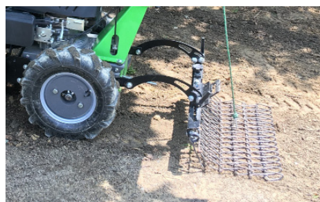
Finishing raking and harrowing
