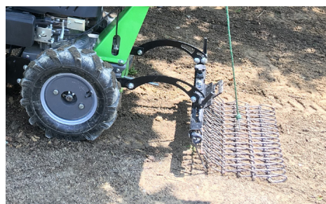
Finishing raking and harrowing
